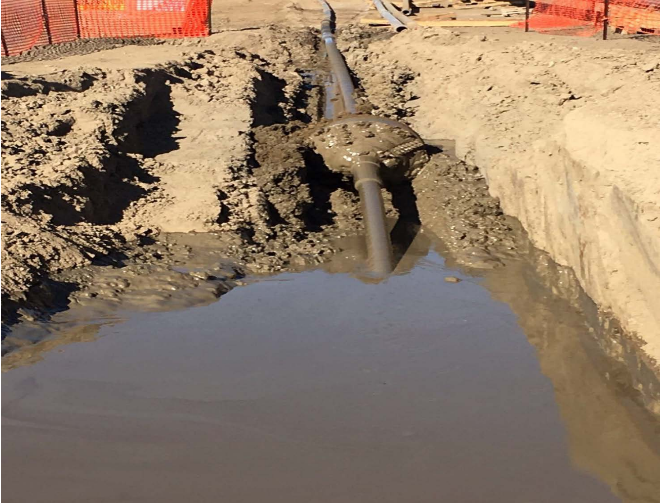
Reamer at Canal Crossing
